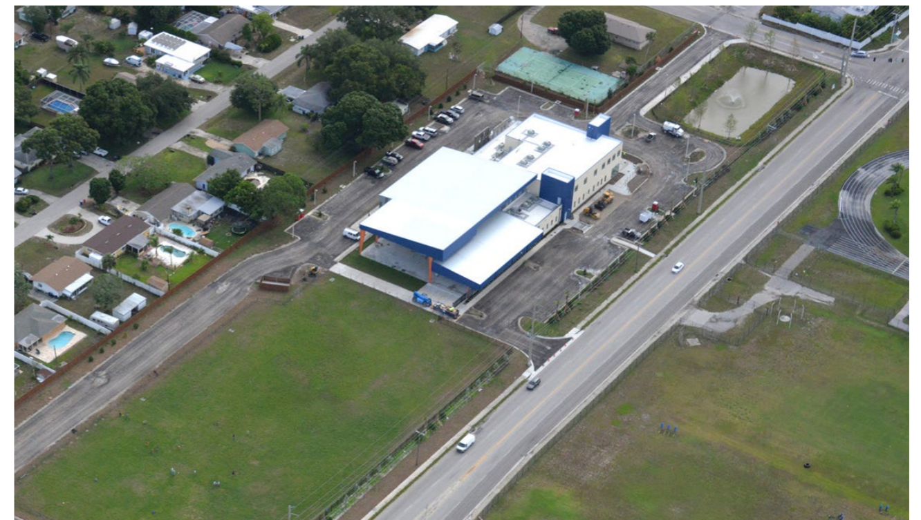
Above: A July 2019 view from overhead and the front of the nearly completed facility
